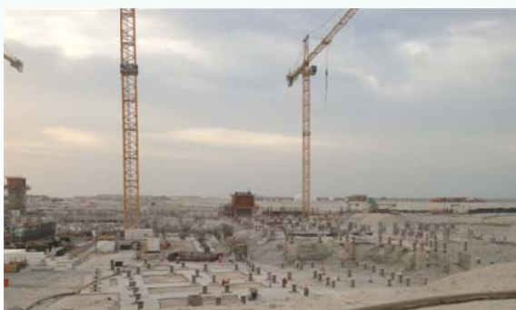
Louvre Abu Dhabi during early construction
