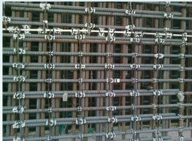
Anodes & conductor bar fixed to rebar clips
