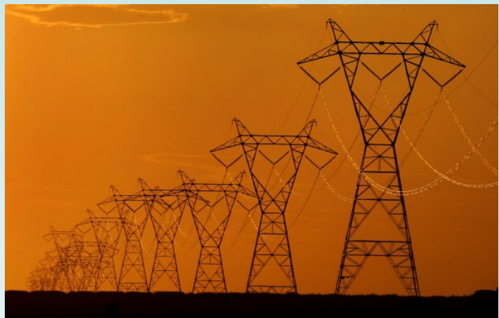
Overhead powerlines can create safety hazards for to personnel working on pipelines
