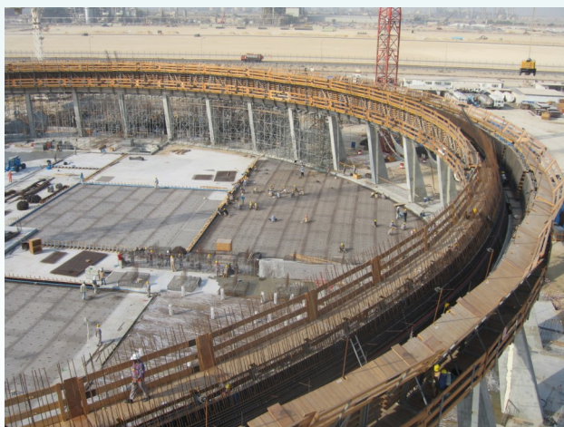
Ring Beam, Columns and CT Shell (first lift)
