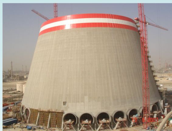
Cooling Tower Near Completion
