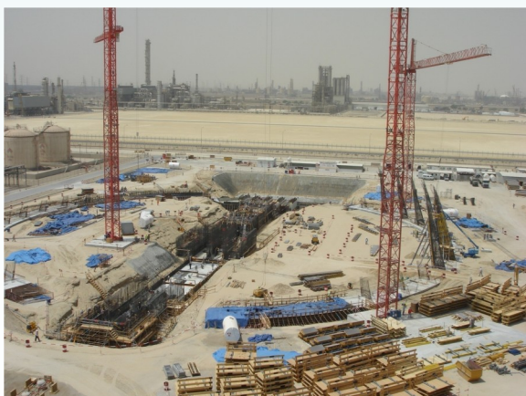
Inlet Duct During Early Construction
