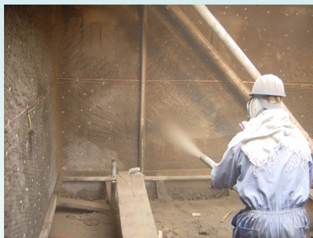
Shotcrete Guniting Over Expanded Mesh
