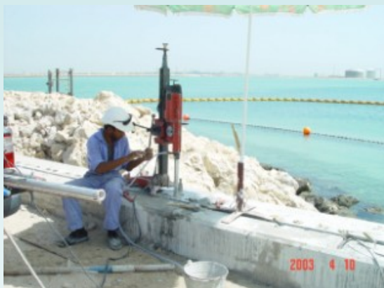
Holes Being Cored in Sea Wall
