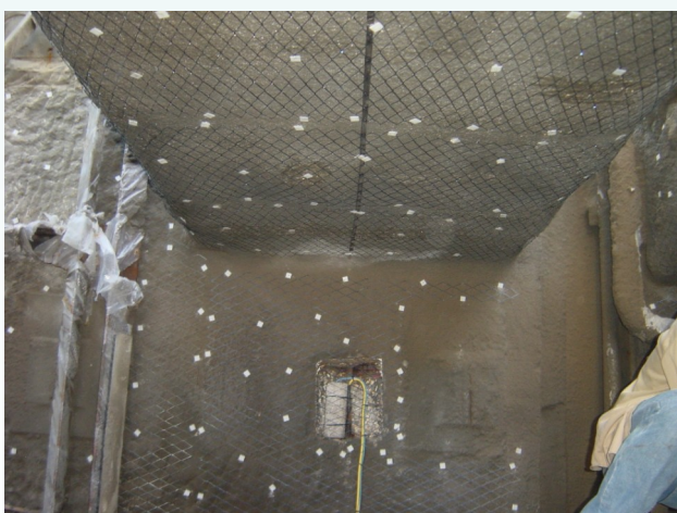
Reference Electrode Installation in Expanded Mesh Wall
