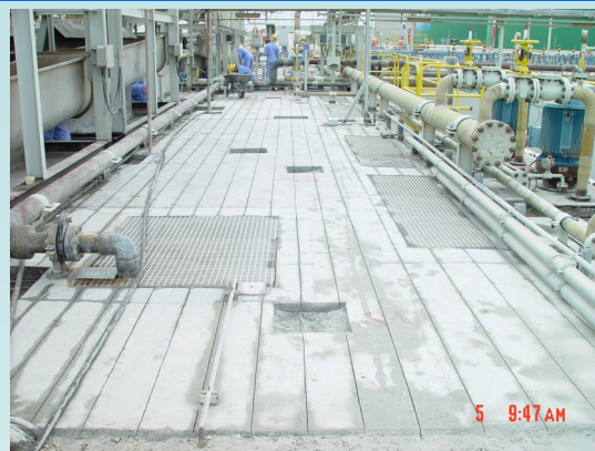
Slotted Anode Installation in Slab
