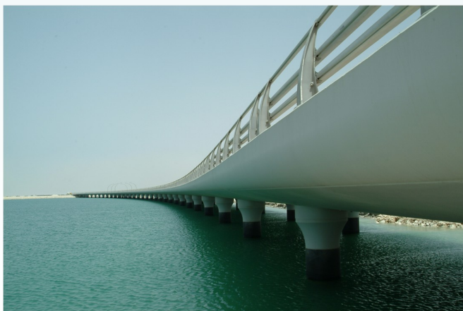
The Elegant Aesthetics of the Bridge
