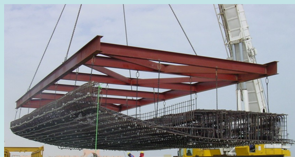
Anode Installation on Bridge Soffit
