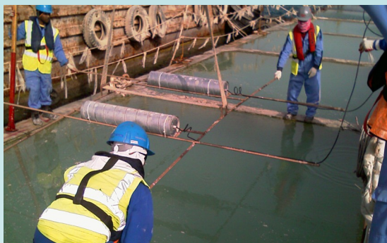
Placement of canistered anodes into a caisson cell
