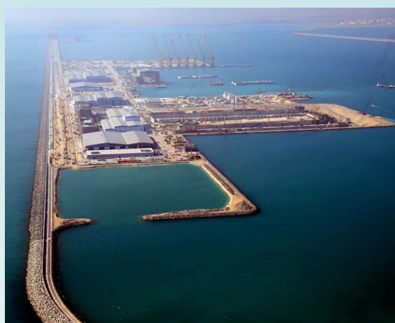
Nakilat Ship Repair Yard (July 2009)
